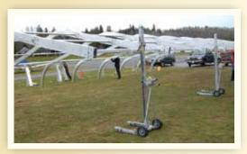
The CAMSS60EX5014 Shelter assembles in sections that slip fit and bolt together. All arches assemble together beginning with the peak. After the peak and ridges have been assembled together, mechanical lifts (included with tool kit) are used to make short lifts to attach eaves and uprights. This slip fit and lift assembly design allows the CAMSS60EX5014 to be assembled without the use of heavy equipment by a crew of six in sixteen hours.
