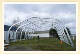
The CAMSS30ISEH48 Shelter assembles in sections that slip fit and bolt together. All arches assemble together beginning with the peak. After the peak and ridges have been assembled together, mechanical lifts (included with tool kit) are used to make short lifts to attach eaves and uprights. This slip fit and lift assembly design allows the CAMSS30ISEH48 to be assembled without the use of heavy equipment by a crew of six in eight hours.
